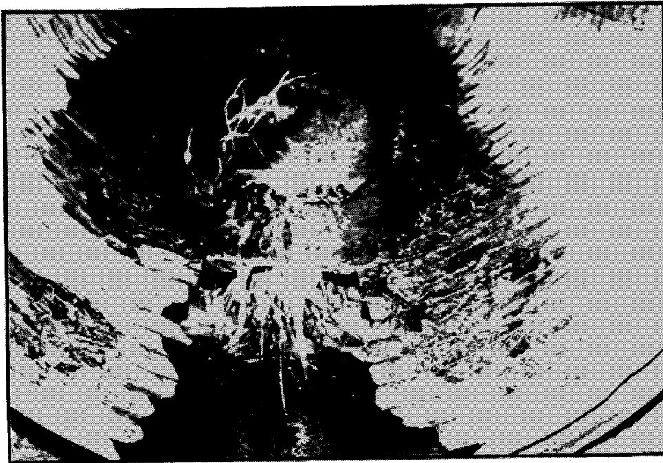
Exhibit 75. Invert deterioration.
