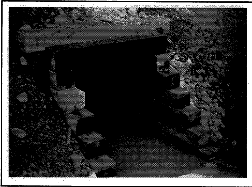
Exhibit 14. Timber culvert. Timber culverts are generally box culverts.
