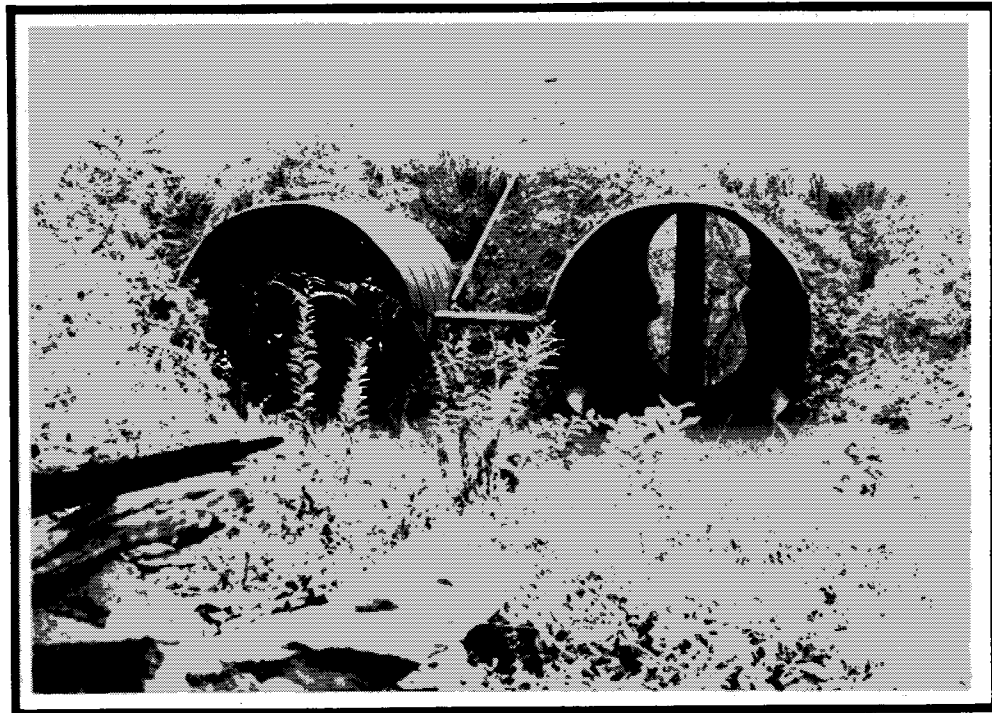
Pipes at same location as top photo require bracing to prevent excessive deflection. Bracing is a temporary measure until permanent repairs can be made.
