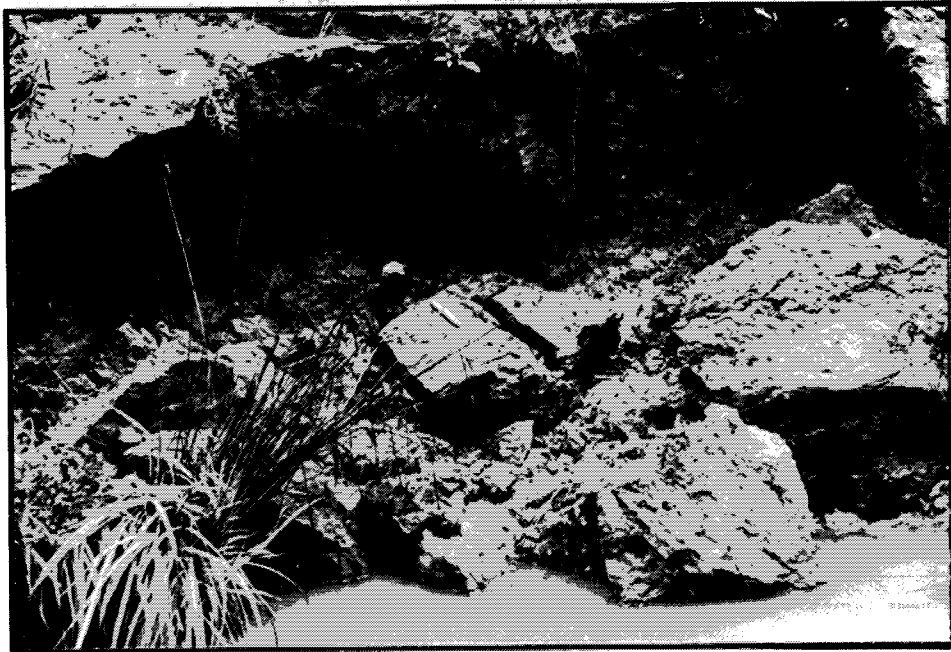
Exhibit 61. Embankment erosion.
